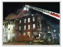
Whiting building destroyed by fire Sunday night
